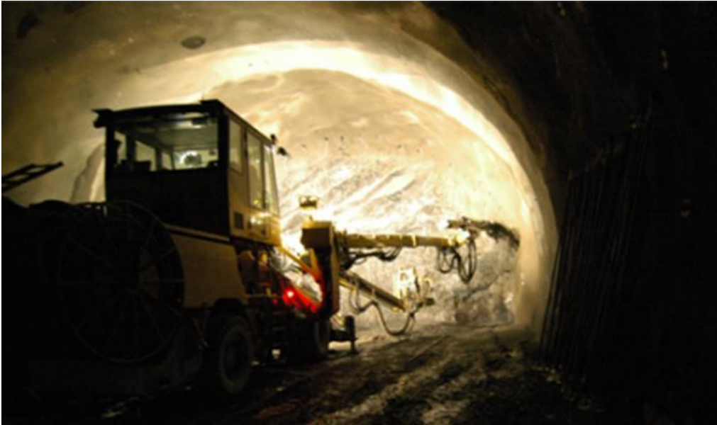
Plate 4.28 Drill and Blast
